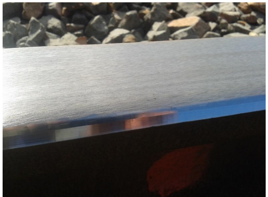
Fig. 3: Example picture of a fully restored rail surface after processing with LINSINGER high performance milling technology.
