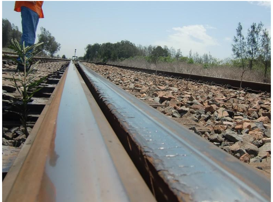
Fig. 4: Surface damages and signs of wear on the profile in the railway track of the bending branch of a switch (ARTC, Australia).
