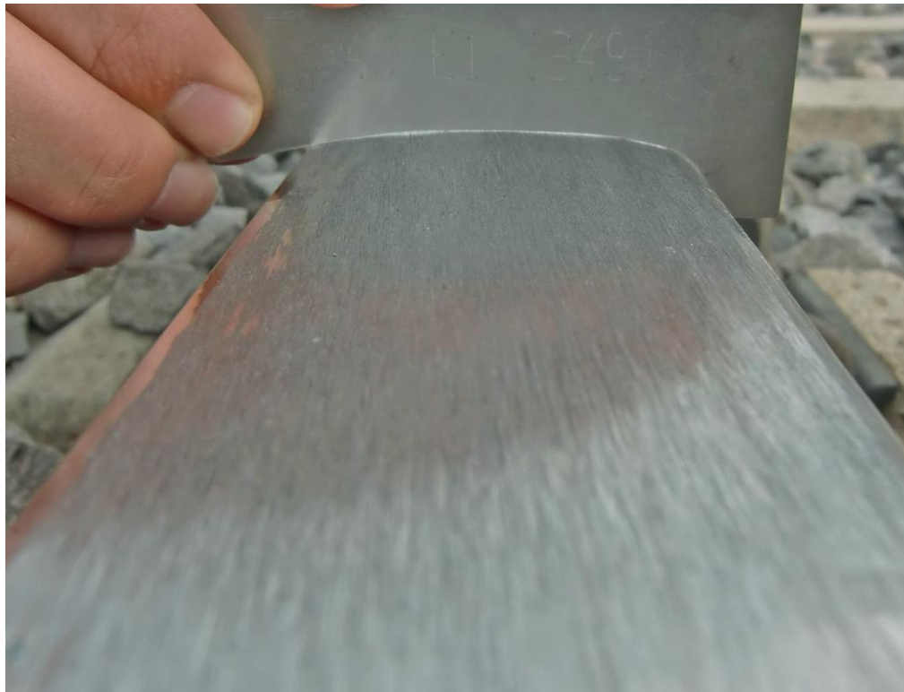
Fig. 2: Rail surface with a perfect surface finish processed with Linsinger high performance milling technology
