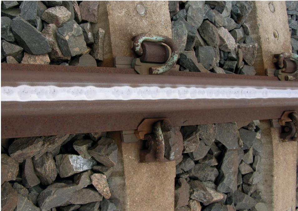
Fig. 4: Squat type defects in multiple occurrences on the railway
