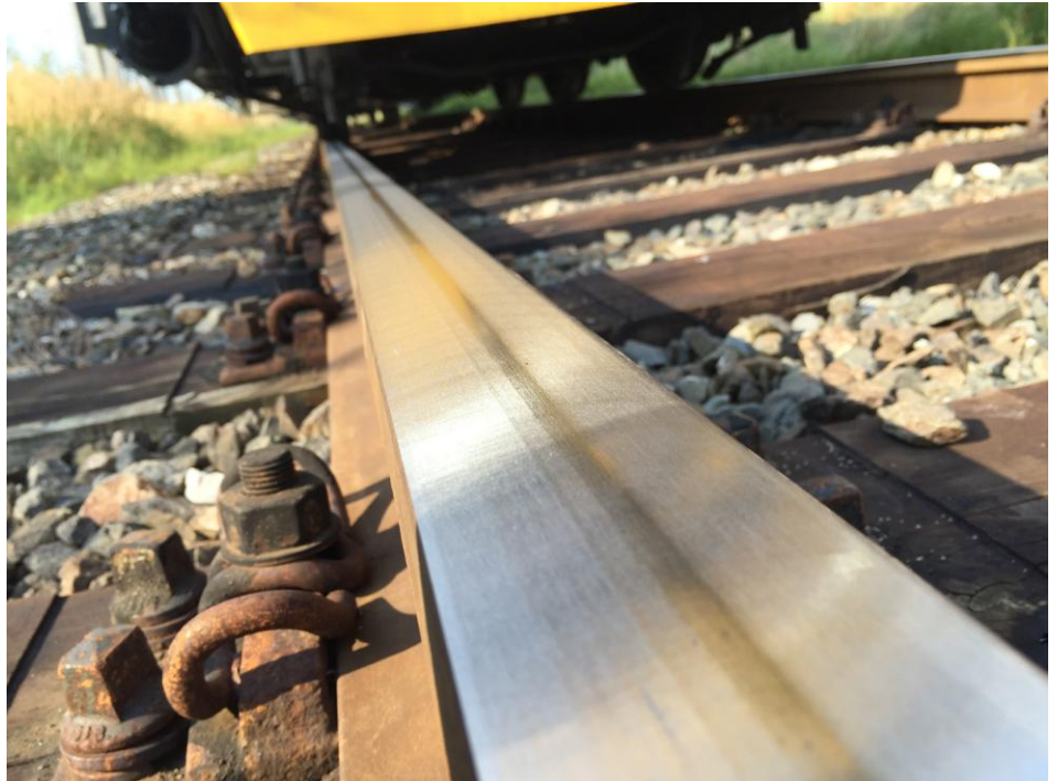
Fig. 1 Rail surface quality after rail milling.
