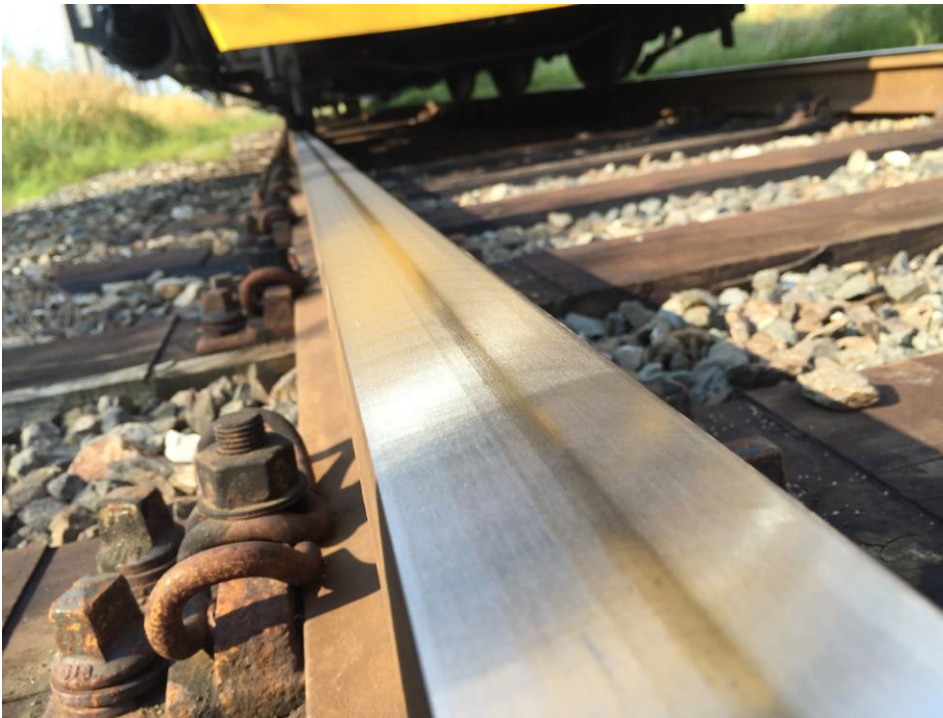
Fig. 2: Usage of Linsinger rail milling machine MG11 at a station in Amsterdam. Dust free processing and without sparks in highest quality.
