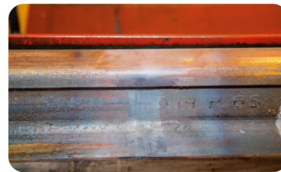
Weld seam after removal
