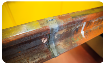
Weld seam prior removal
